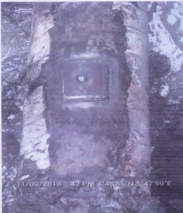
REPAIRED SPILL POINT.
