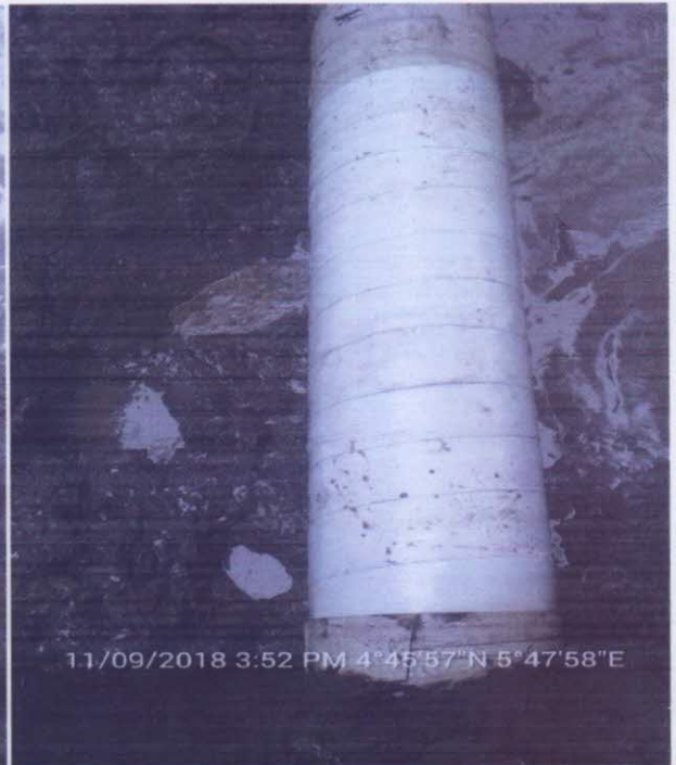
REPAIRED AND WRAPPED.
